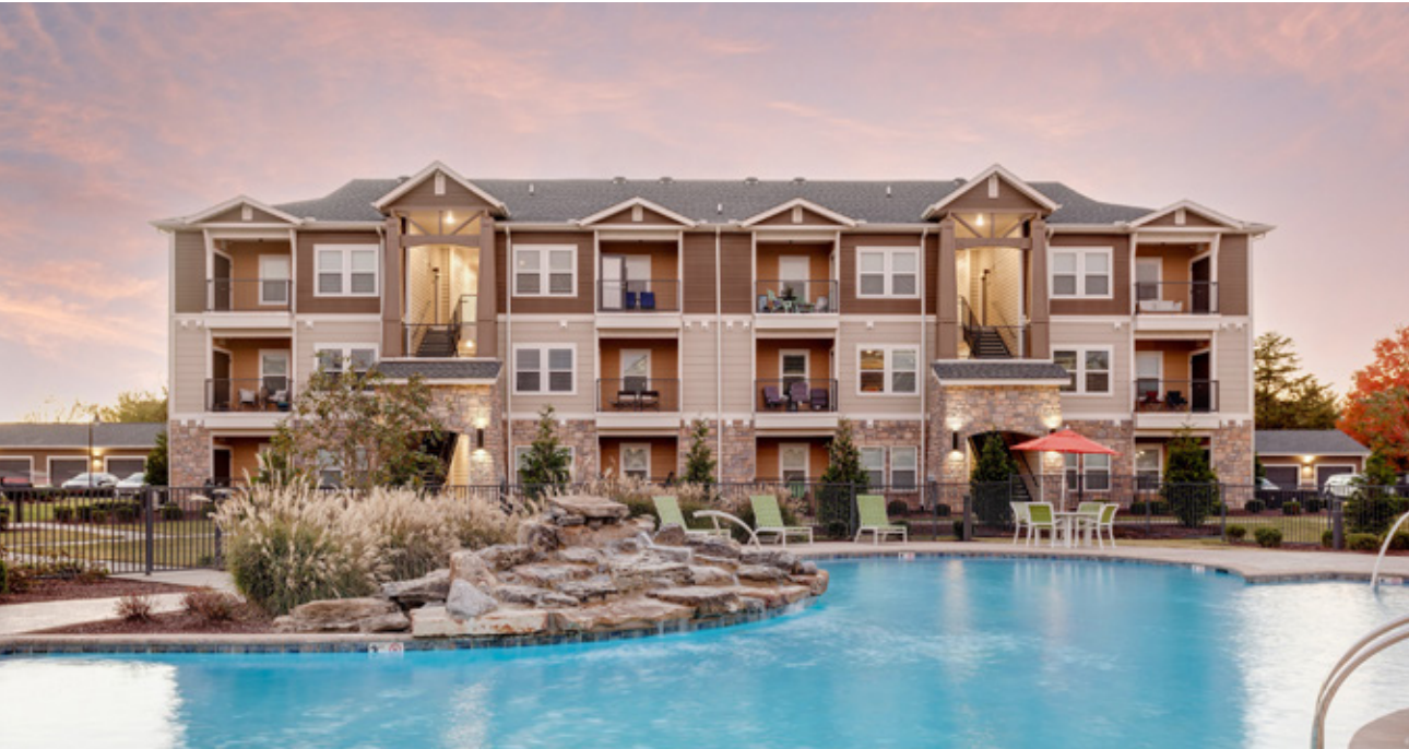
THE EDGE, multi-residential building Real estate | Tennessee, United States | Partner: BGO
