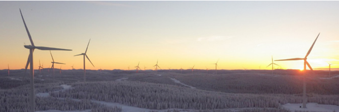
RIVIÈRE-DU-MOULIN WIND FARM Quebec City, Canada Partner: EDF Renewables Photo credit: Joan Sullivan
